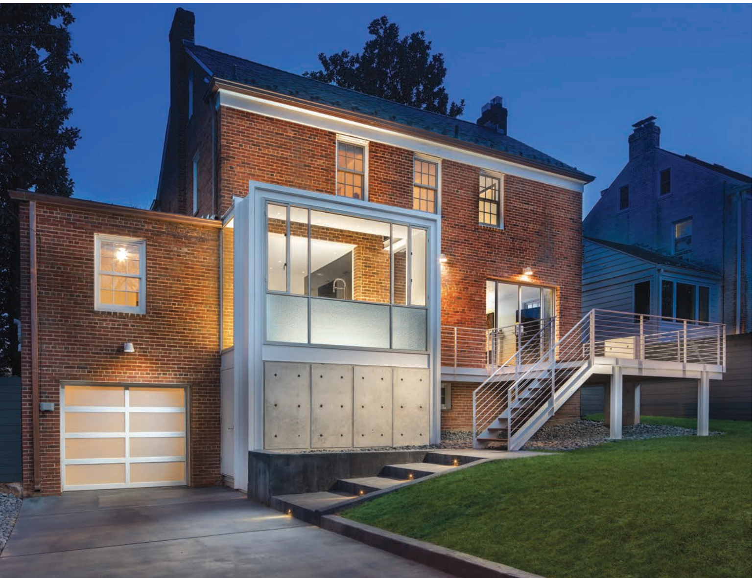
Rear of the Fessenden Street house following renovation, showing the new bay of the kitchen at left center with storage below, and the new deck at right.
